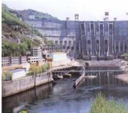
Figure 5.1: Baishan Hydropower Station.
